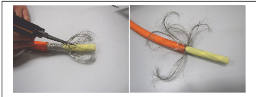
Fig. 6-6: Split the shield braid open
